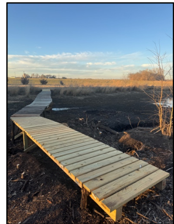
Newly constructed island bridge (Thanks Calvin & Henry Janzen)
